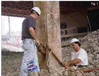
Fig.1 Demolition engineers at work – note diagonal angle of explosive cutting charge.
