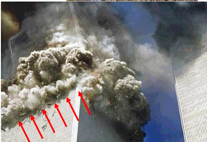
'Squibs' — a neat row of cutter charges exploding, before dust obscures progressive demolition.
