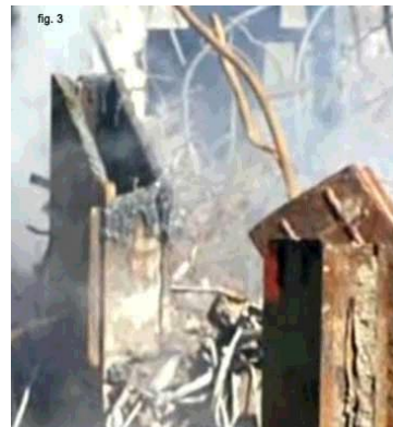
'Cut' metal beams at base of WTC. Note the steel edge was melted, denoting the use of thermate steel-cutting demolition explosive. Compare diagonal angle in Fig 1.
