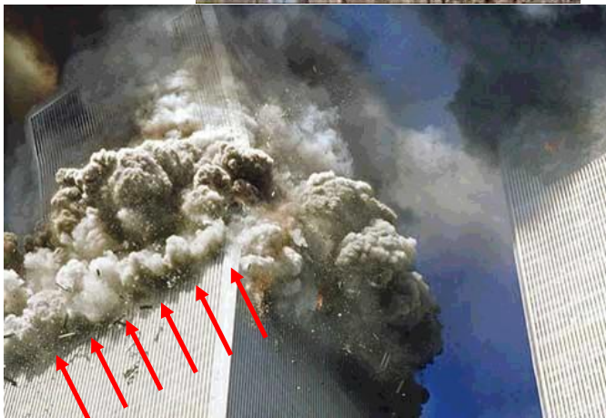
'Squibs' — a neat row of cutter charges exploding, before dust obscures progressive demolition.
